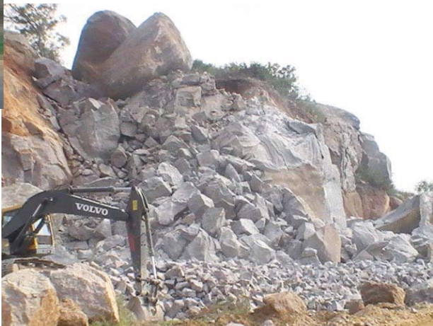
Brahma Rock on Outer Ring Road - Destroyed
